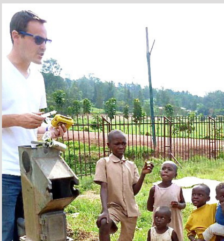
Evan Thomas replacing a wireless transmitter in a water pump, as young users look on.
